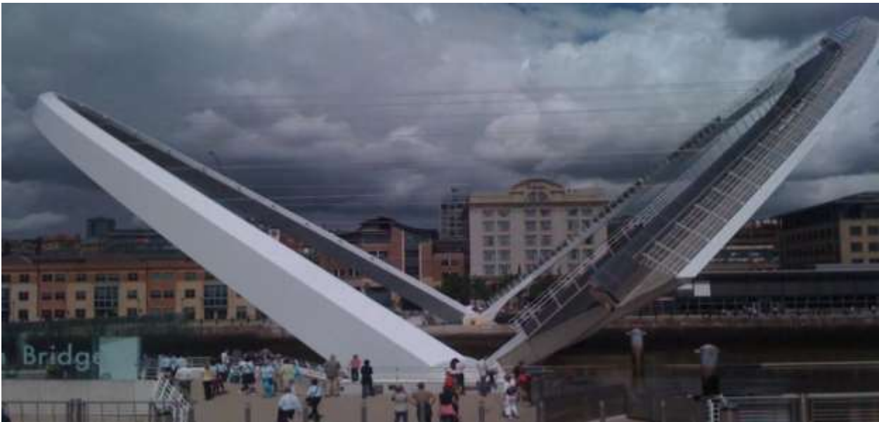
Figure 29: Illustration of an open tilt bridge (Gateshead Millennium Bridge, photograph by Hewson Engineering)
