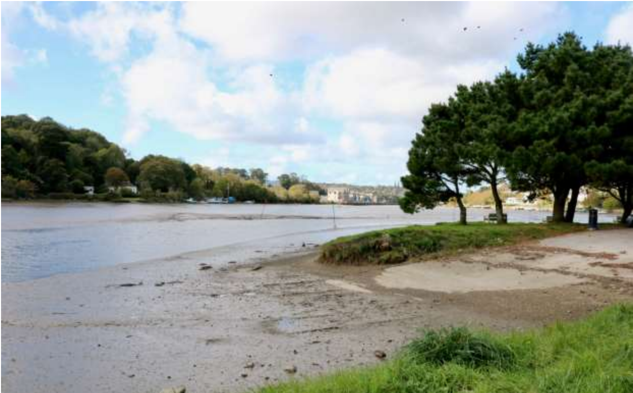
Project 8 – Existing slipway and level of silting up
