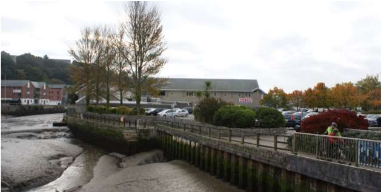
Project 4 – Current condition of link between city and river
