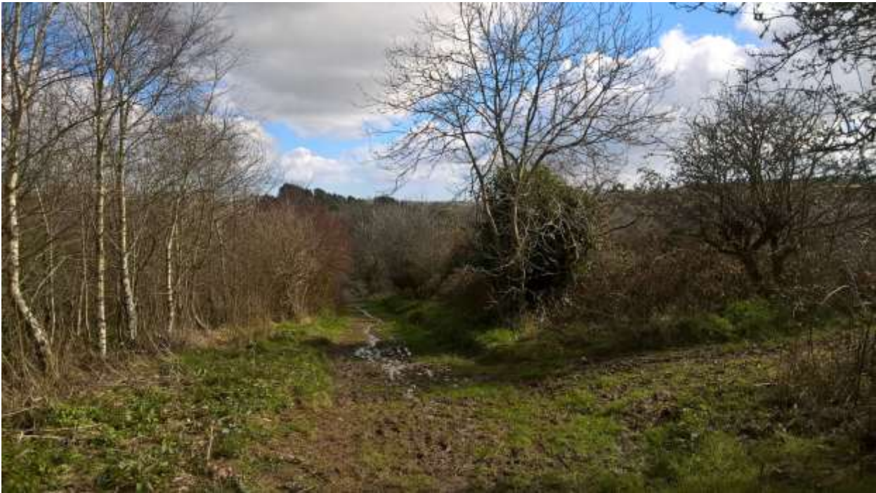
Project 14 – Current condition of new link shown for Moresk Forest area, will require some improvement to be usable for cycling
