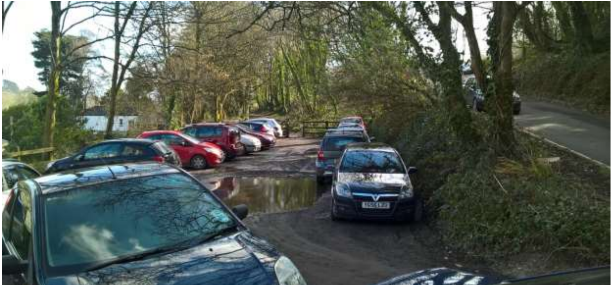
Project 9 – Condition of existing car park for improvement
