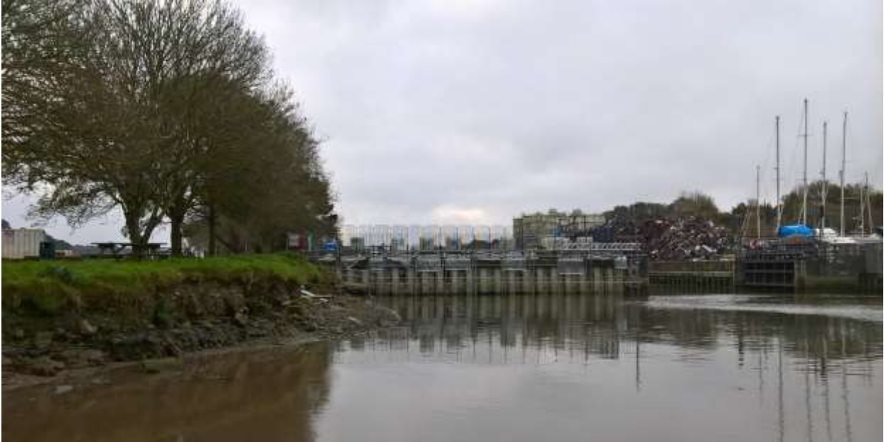
Project 2a – Floodgates and Boscawen Park edge – bridge would be in front of the floodgates in this view
