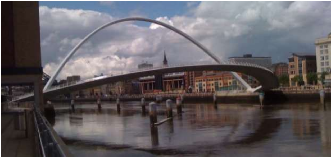
Figure 28: Illustration of a tilt bridge in a lowered state (Gateshead Millennium Bridge, photograph by Hewson Engineering)
